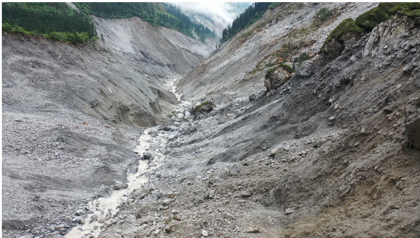
Landslide of Bhemathnag at the top of Melamchi River in Sindhupalchowk. Photo: Vikash Lamsal
